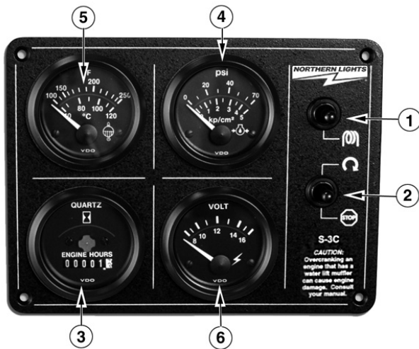
Figure 6: Series 3 Generator Control Panel
